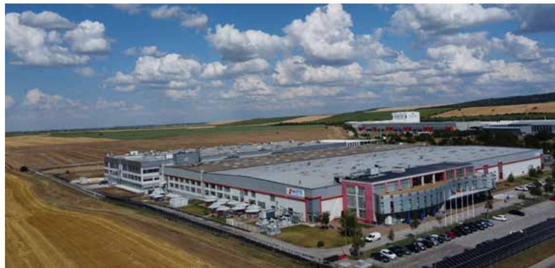
Exterior view of the Ruse plant
