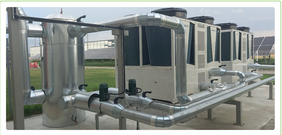
Heat pump cascade and photovoltaic modules in Ruse
